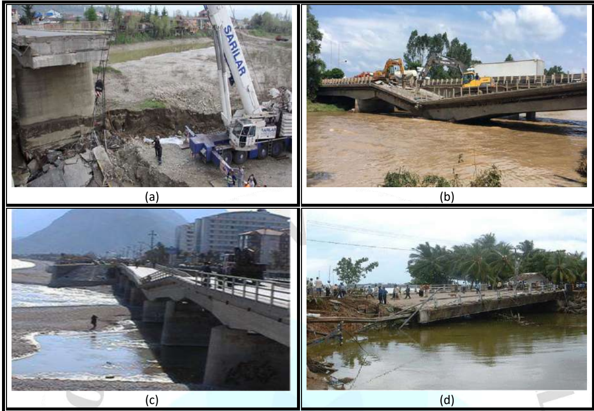
Figure 1. Examples of bridge damages and collapses (Zaky, 2019): a) Post-flood state of the bridge in Çaycuma district of Zonguldak province in Turkey; b) Condition of Cevizdere bridge after flood in Ünye district of Ordu province in Turkey c) Boğaçay bridge damaged appearance; d) Magalle bridge in South of Galle, which was destroyed due to the pierced pit.
