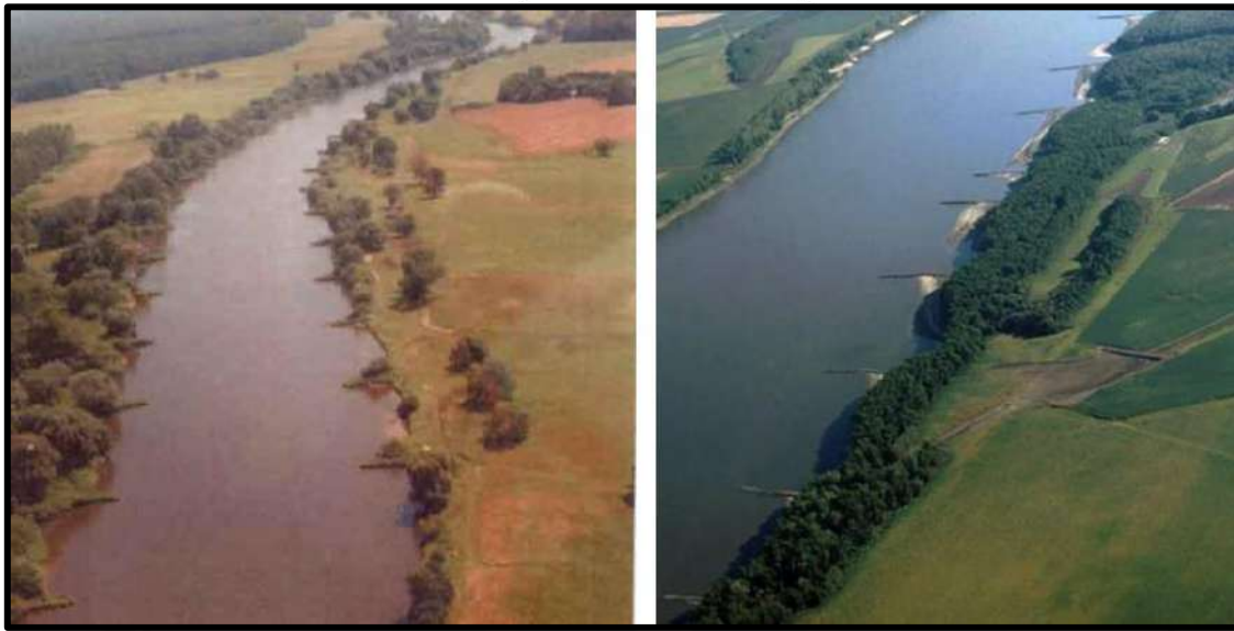
Figure 1. Bidirectional and unidirectional spur applications a) Odra River (Poland) b) Mississippi river (USA) (Özyaman, 2016)
